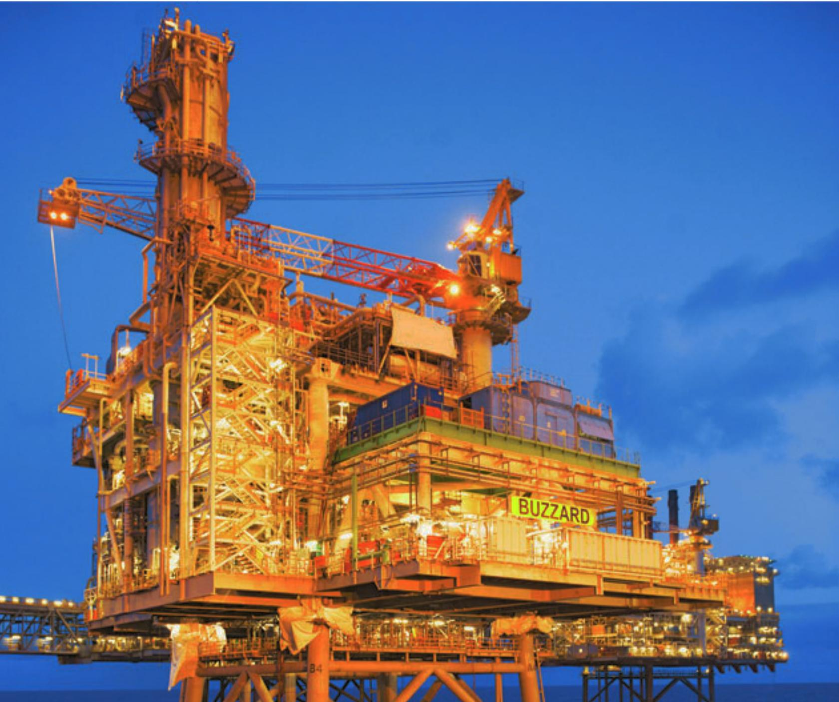
The 2010 installation of a production sweetening facility has enhanced Nexen's ability to process naturally occurring hydrogen sulphide in the oil produced from our Buzzard platform, offshore United Kingdom.
