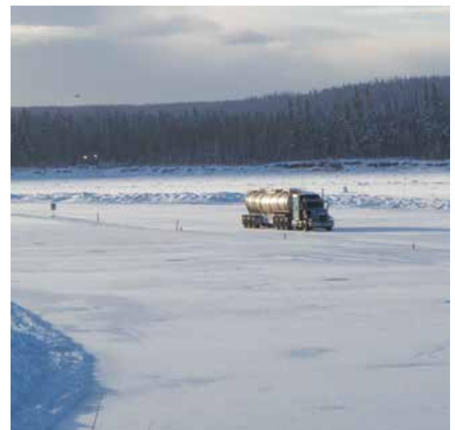
Semi-truck delivers materials over Liard River ice bridge. The bridge is 1.5 kilometres long – 750 metres of travel is on gravel and 800 metres on ice.
